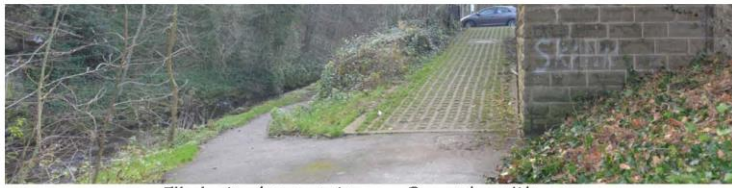
View 3 Eliminate adverse camber and provide upstand kerb edge and possible handrail Proposed possible access ramp [DDA compliant??]
